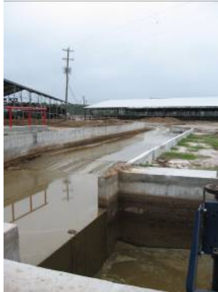
Plate 1. Passive Channel Sand Separator
