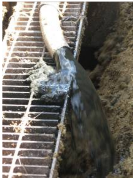
Plate 3. Return of thickened sludge from TFS mixing the coarse solids
